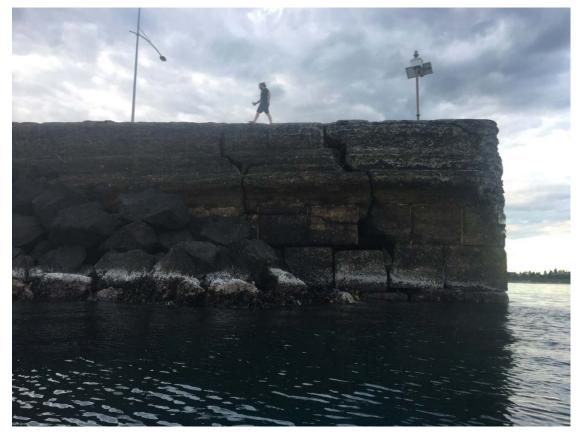
Figure 11 Armour Rocks at Breakwater Head
