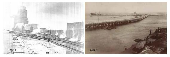
Figure 1 Warrnambool Breakwater construction circa 1890 and completed Breakwater in early 1900's
