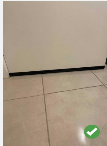
Figure 5: Post-installation photo showing weather seal on bottom of door
