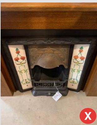
Figure 7: Canopy style interwar period fireplace with a metal damper that only partially seals – front view
