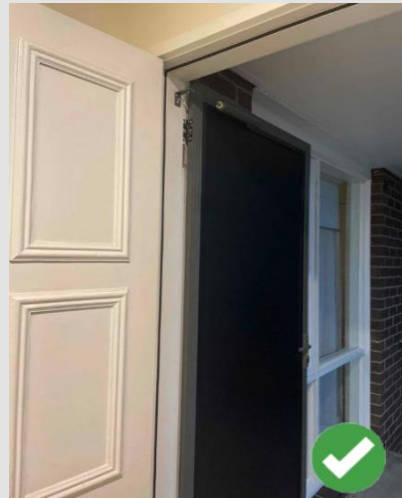
Figure 3: Post-installation photo showing weather seals on two sides of door frame
