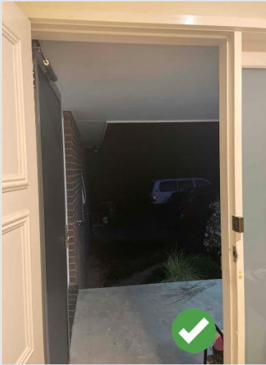
Figure 2: Photo showing the entire perimeter of the door, demonstrating it is an external door
