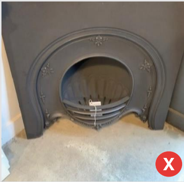
Figure 3 Less common Victorian style where the damper is held with a ratchet mechanism – front view
