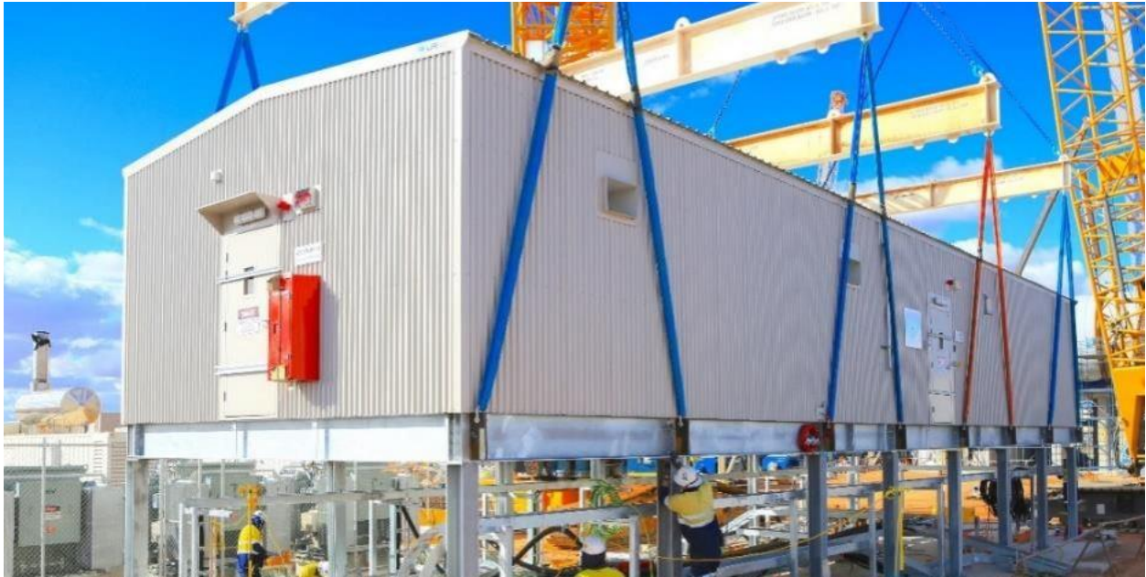
Figure 3 Control Room Example
